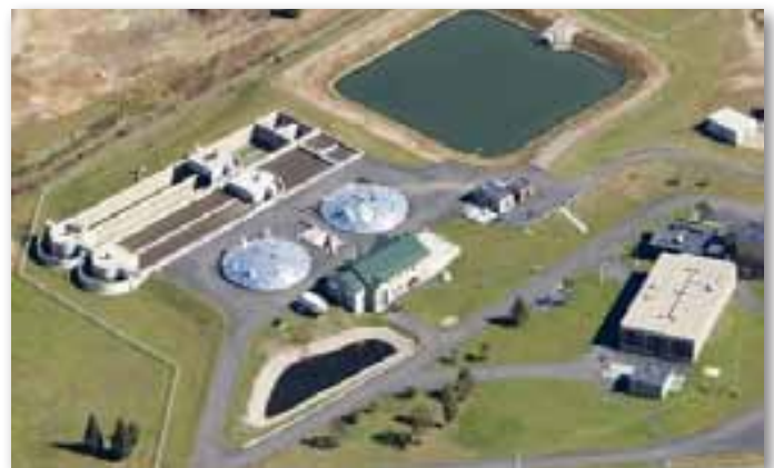
Sanford, ME Wastewater Facility uses both biological and chemical removal strategies to convert soluble phosphorus to insoluble phosphorus. The suspended phosphorus is removed with flocculation, lamella clarifiers, and sand filtration to achieve a phosphorous limit of 0.1 mg/l.
