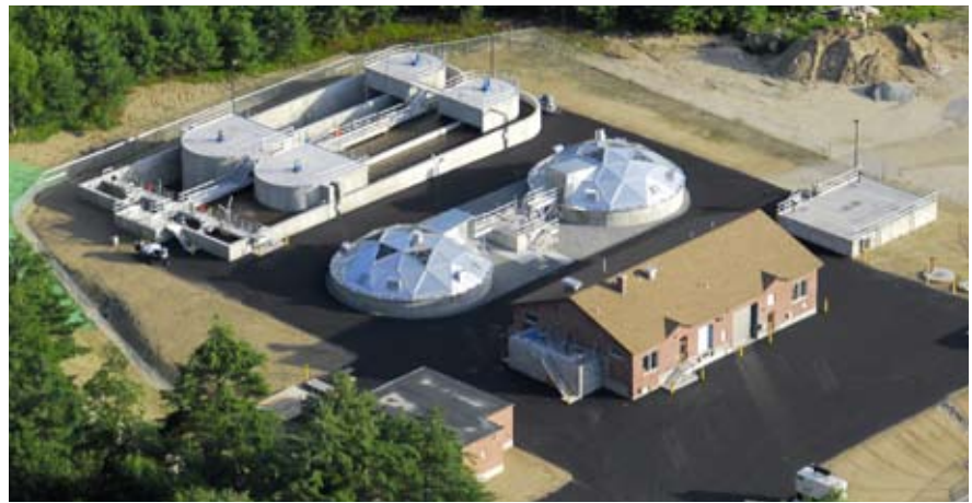
There are many BNR process configurations available. The best option for a given facility is case-specific and depends on various factors, including effluent standards, waste characteristics, site constraints, etc.
